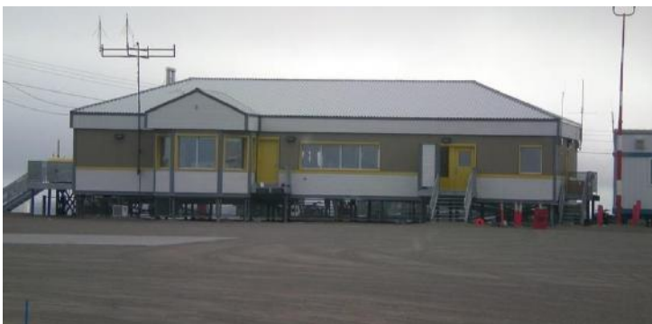
Gjoa Haven's airport
